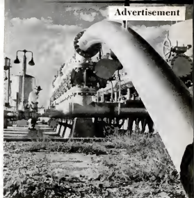
MODERN PIPELINES , like this 12-inch line at Hearne, Texas, cut transportation costs, help refineries meet competitive prices. If North Dakota's oil hopes are realized, vast new pipe-line facilities will be needed to transport the oil to other parts of the country.
