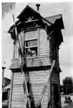
IN TOWER Herb recalls the tale of a crossing where trains snuck by.
