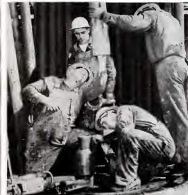
OIL DRILLING CREW sets pipe. Record deep-drilling operation, in Mississippi, is nearing 4 mile depth. Sharp competition in U. S. oil fields results in world's best drilling methods.
